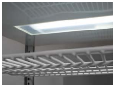
Internal lighting in the ceiling
